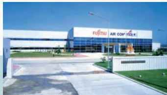
Fujitsu General (Thailand) Co., Ltd. Fujitsu General Engineering (Thailand) Co., Ltd.
