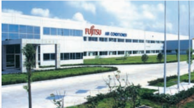
Fujitsu General (Shanghai) Co., Ltd.
