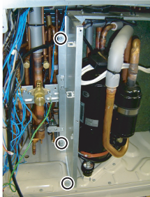
Remove the 3 mounting screws.
