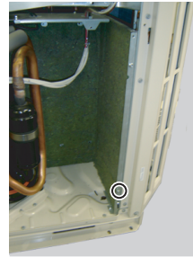
Remove the mounting screw.
